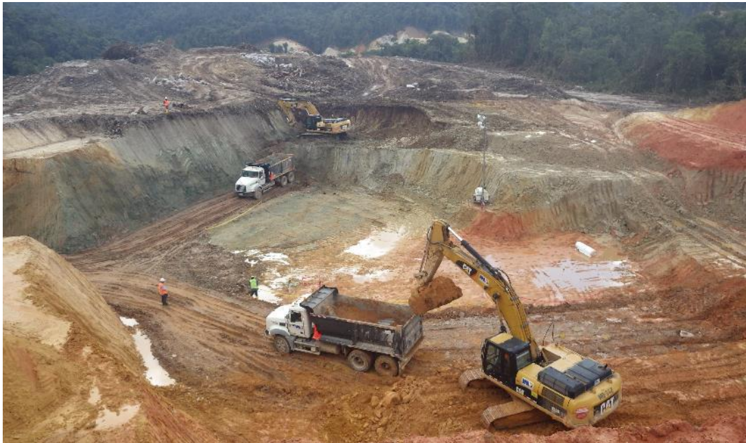
Figure 2. Process plant earthworks
