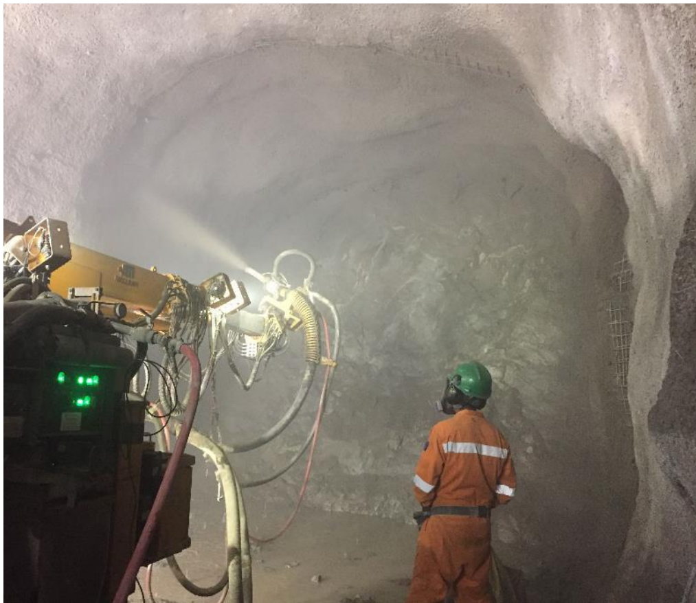
Figure 1. Hard rock tunneling at Fruta del Norte underground mine
