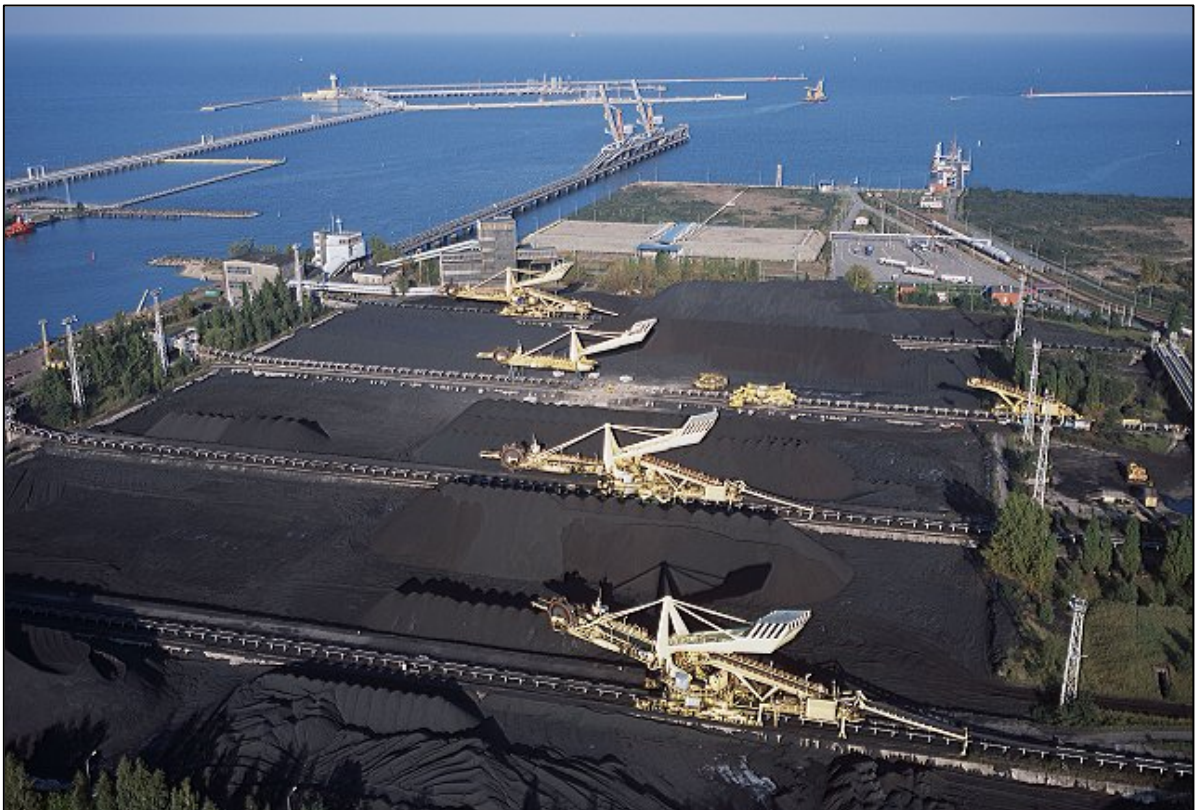
Figure 7: Gdansk Port – “Dry Bulk Terminal” – export facility stacker/ reclaimers
