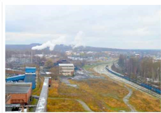
Figure 3 – Existing Site Facilities
