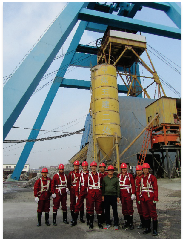
Figure 1 – Prairie Mining team visit CC5C shaft sinking site in China
