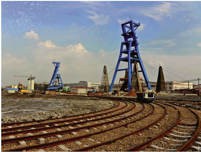
Figure 6 – Auxiliary Shaft at Zhangzhuang Iron Mine
