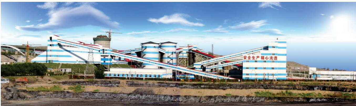
Figure 8 – 22 Mtpa Coal Wash Plant developed and constructed by CC5C
