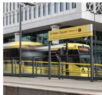
VixTech – Manchester Metrolink platform
