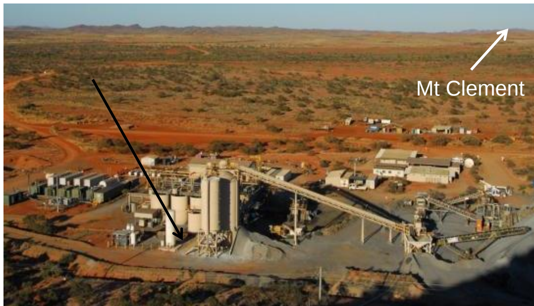
Paulsens CIP Plant ~30km from Mt Clement (Owned by 20% JV partner Northern Star Resources Ltd)
