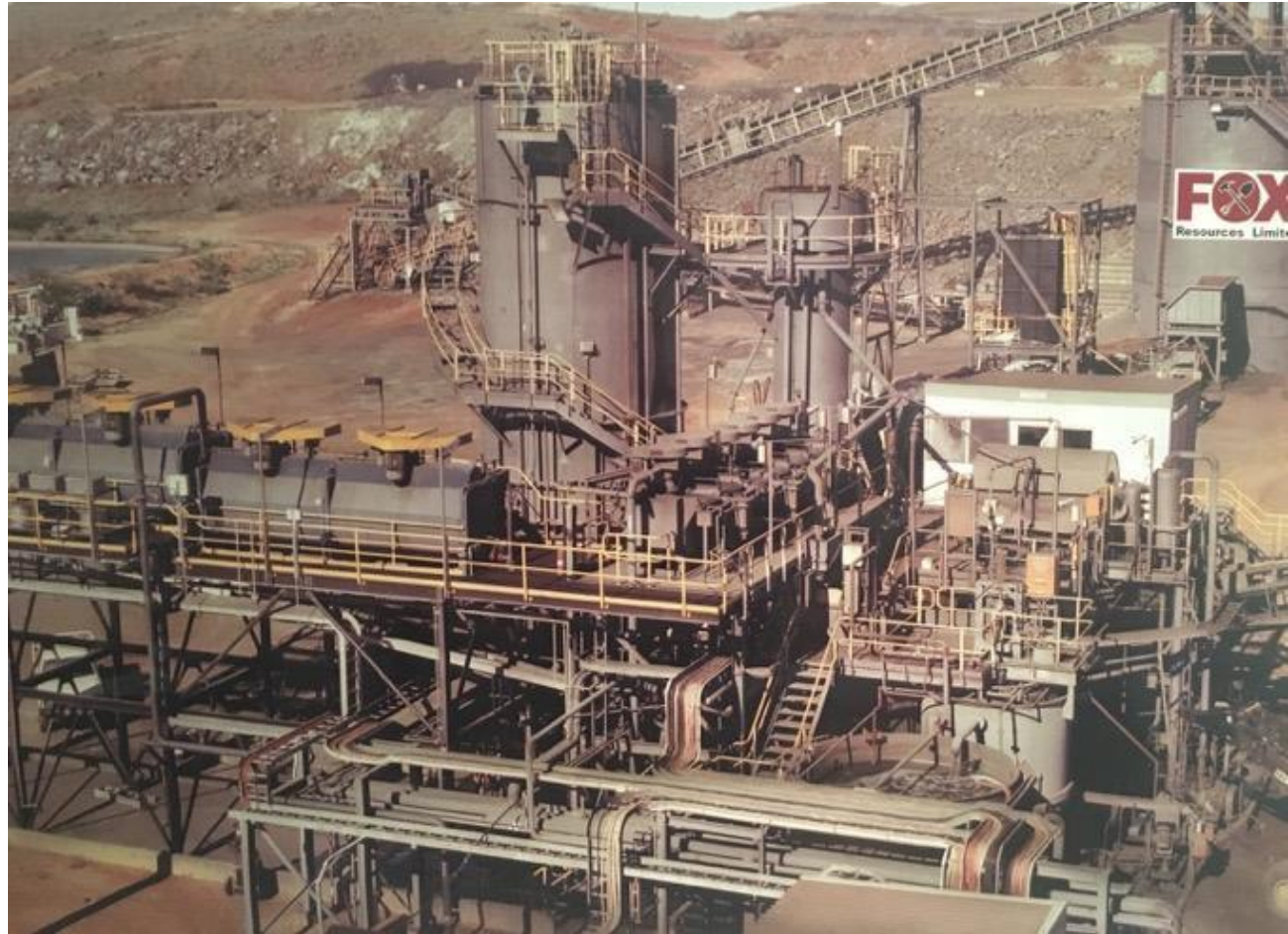
425,000 tpa Radio Hill Treatment Plant – Karratha, WA
