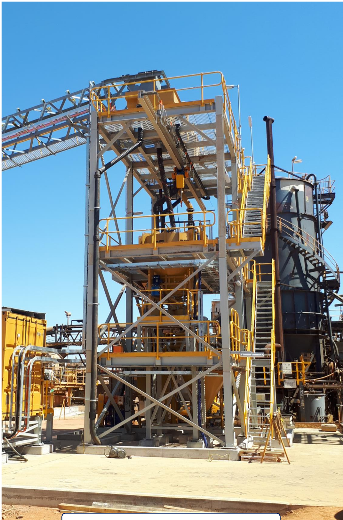
Figure 2 – Gravity Concentrator Tower
