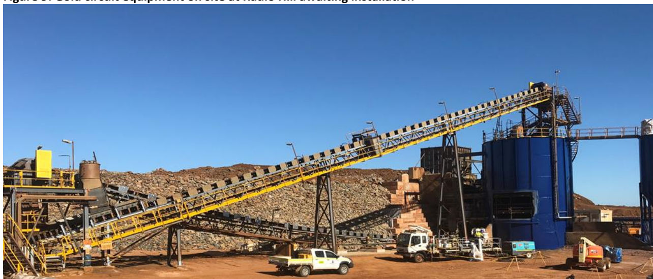
Figure 10: Refurbished crushing circuit and fine ore bin
