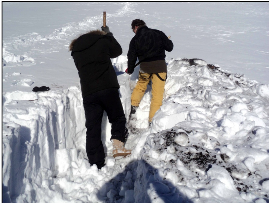
Figure 5-10: Clearing the snow from a trench
