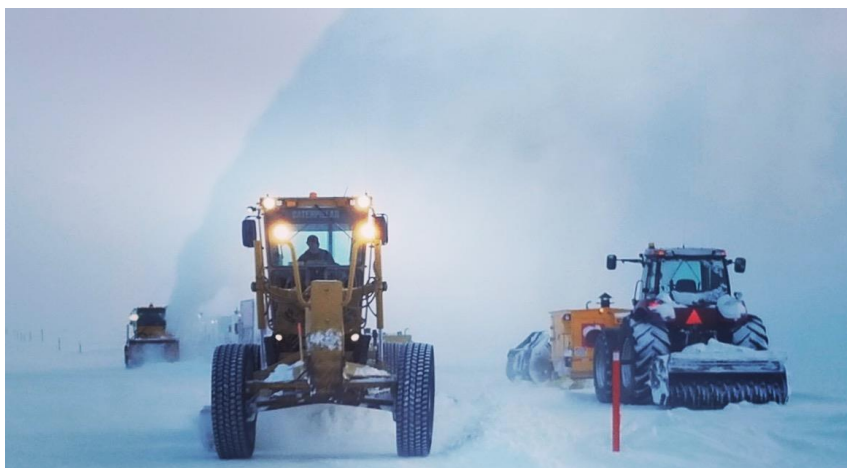
Figure 1 | Ice road construction.
