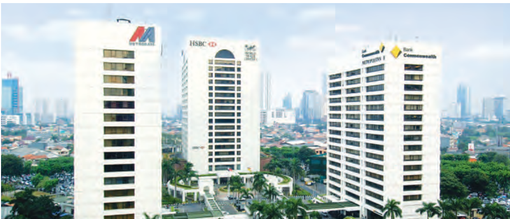
Jakarta Land – Wisma Metropolitan I & II and WTC I
