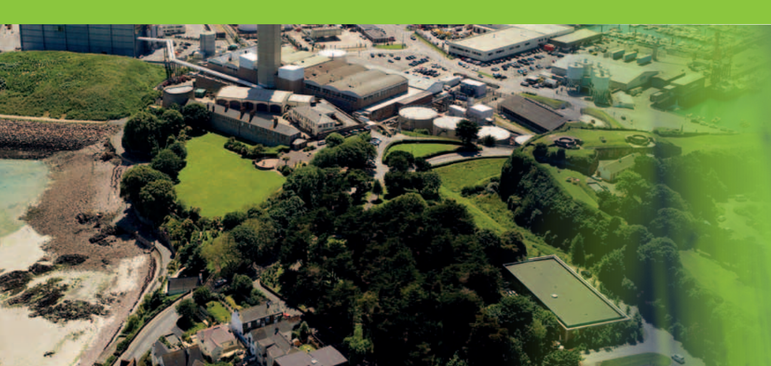
South Hill Switching Station
