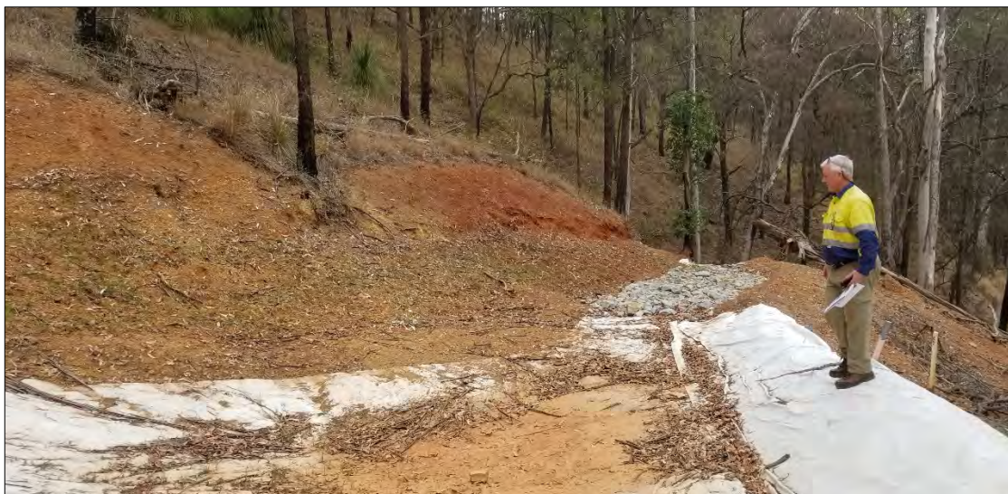
Figure 3-26 Photograph of a settling pond and lined drainage channel installed to manage rainwater run-off from drilling pads and access tracks (SRK ES Sept 2019)
