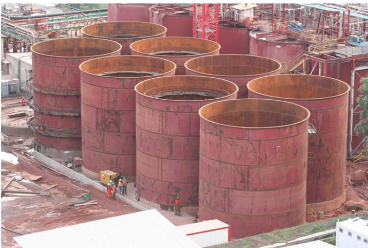
Figure 2. Oxide CIL tank erection October 2013
