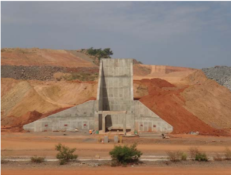
Figure 1. Completed Oxide crusher structure - October 2013
