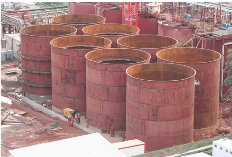
Figure 2. Oxide CIL tank erection October 2013
