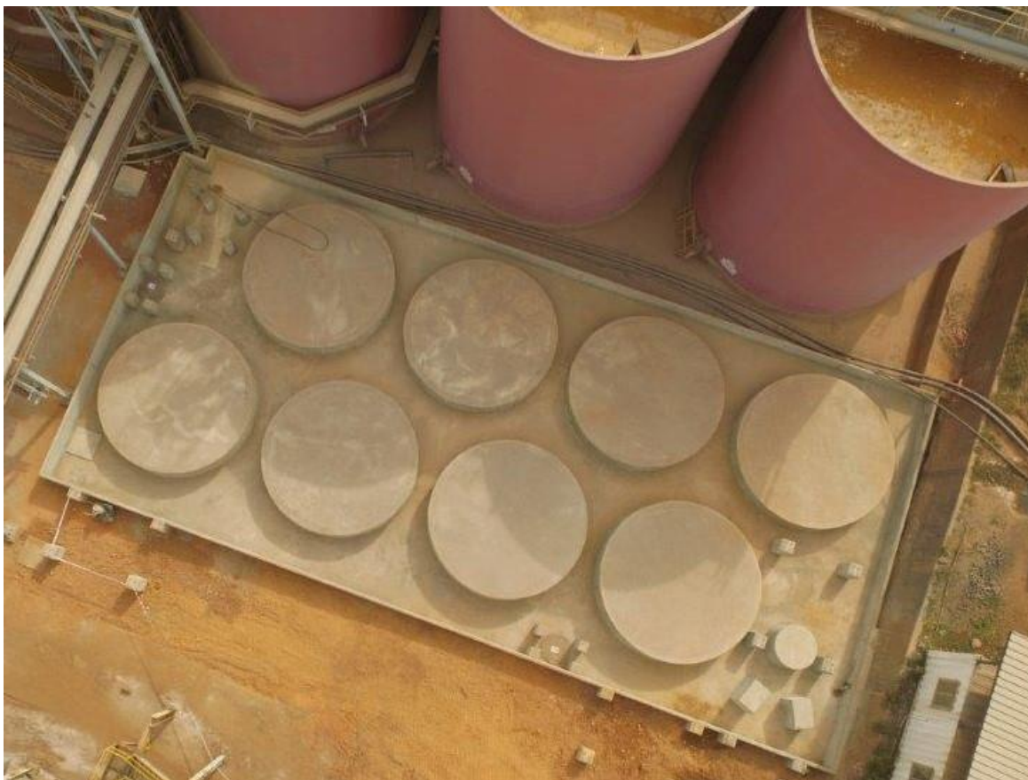
Figure 4: Syama Project 85 site civil work completed
