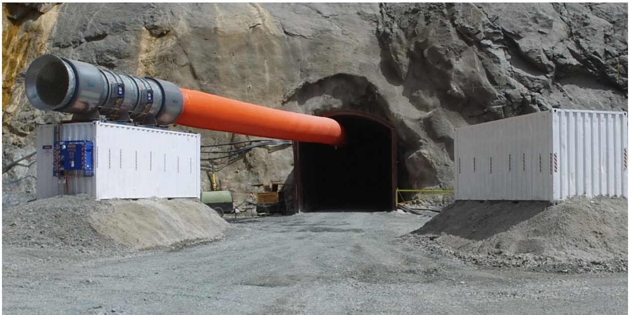
Figure 3: Syama Underground 1200 portal established
