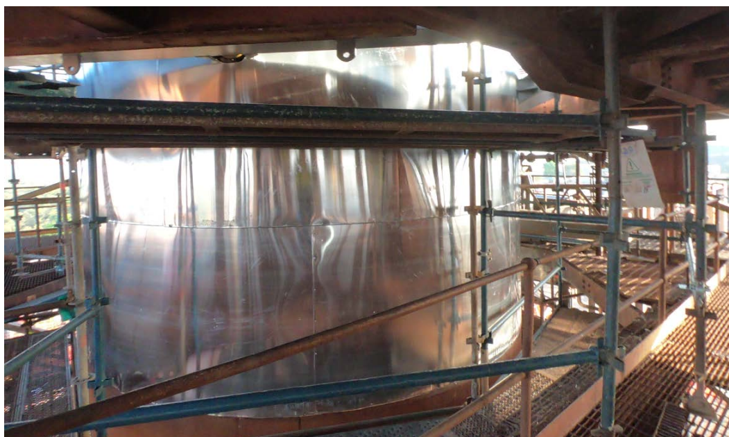
Figure 3: Syama Roaster repair completion
