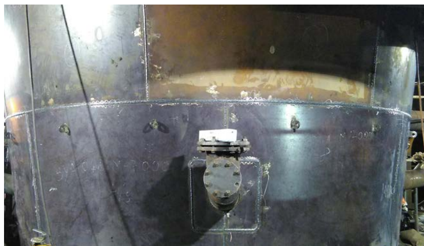
Figure 2: Syama Roaster steel replating
