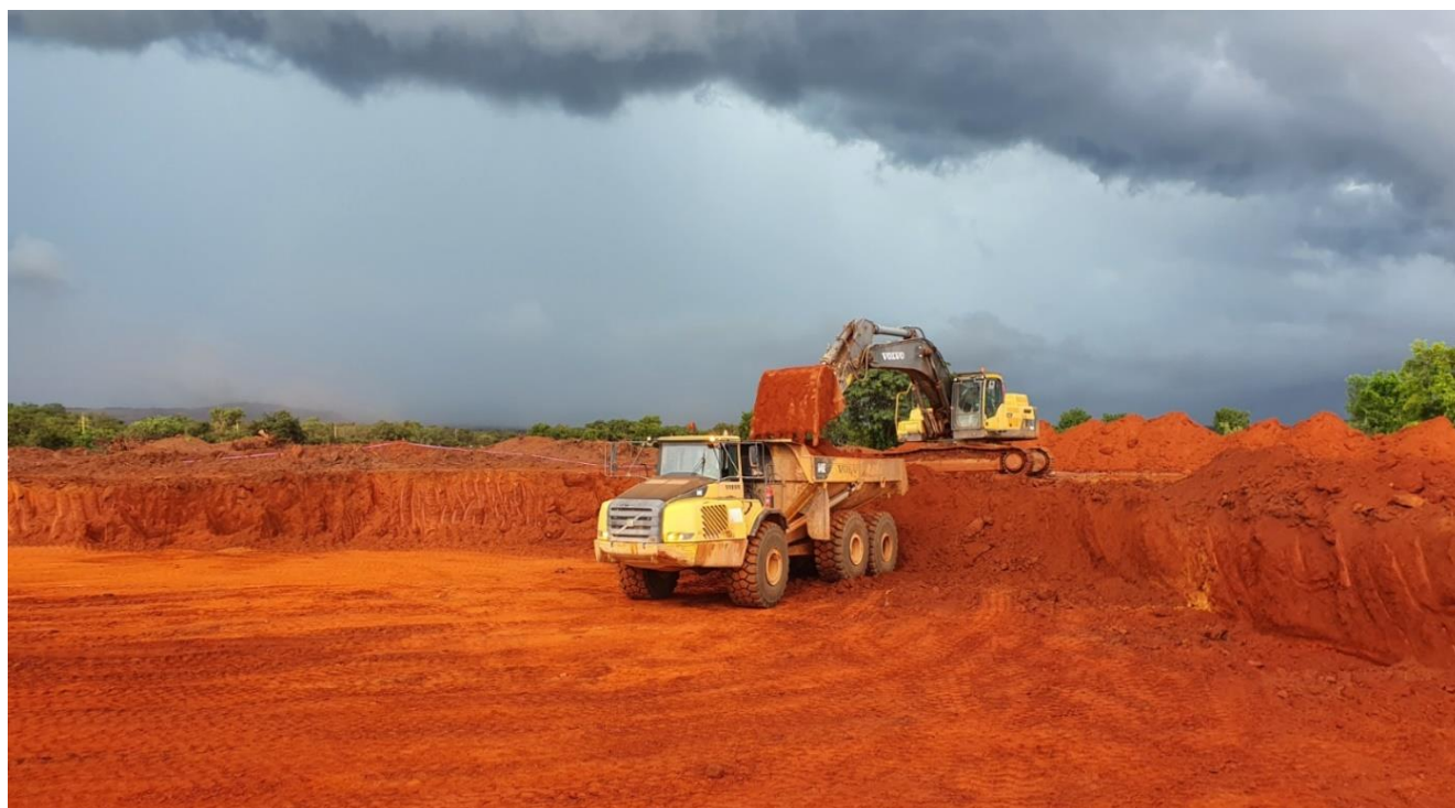
Figure 1: Establishment works at the Cashew mining operation
