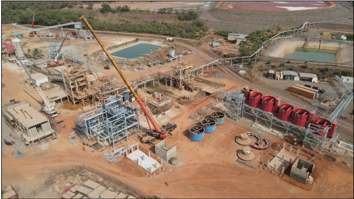
Figure 1: Ball mill and flotation areas in December under construction. The flotation circuit is now 50% complete, while the ball mill areas is 30% complete
