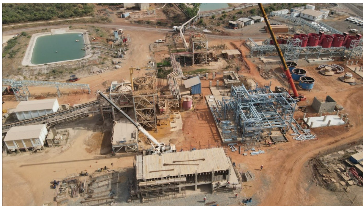
Figure 3: The milling area substation is 15% complete
