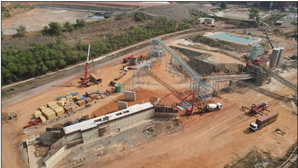
Figure 2: Secondary crusher and sulphide stockpile feed conveyor areas are 35% and 10% complete respectively
