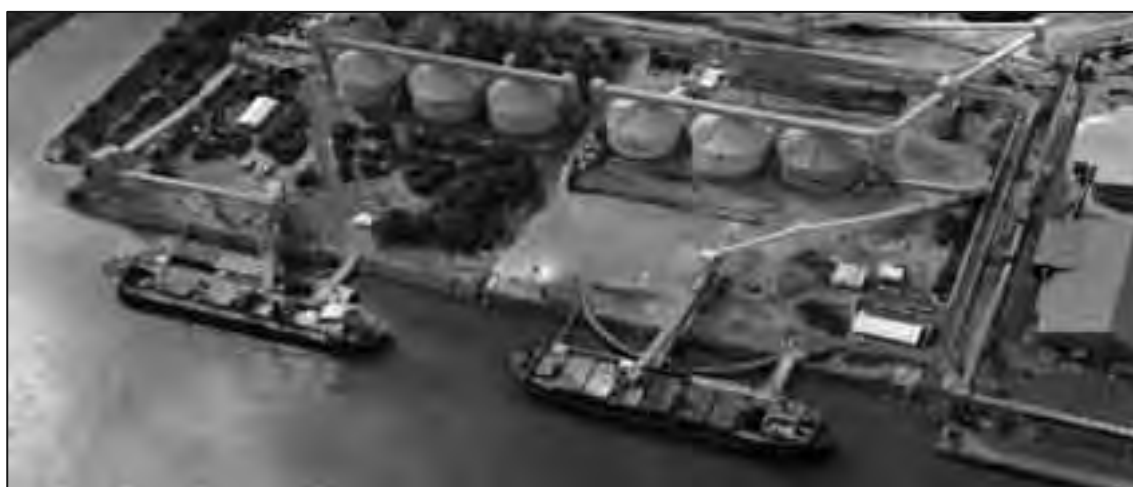
Figure 9-2: Worsley Alumina port facility (right side)
