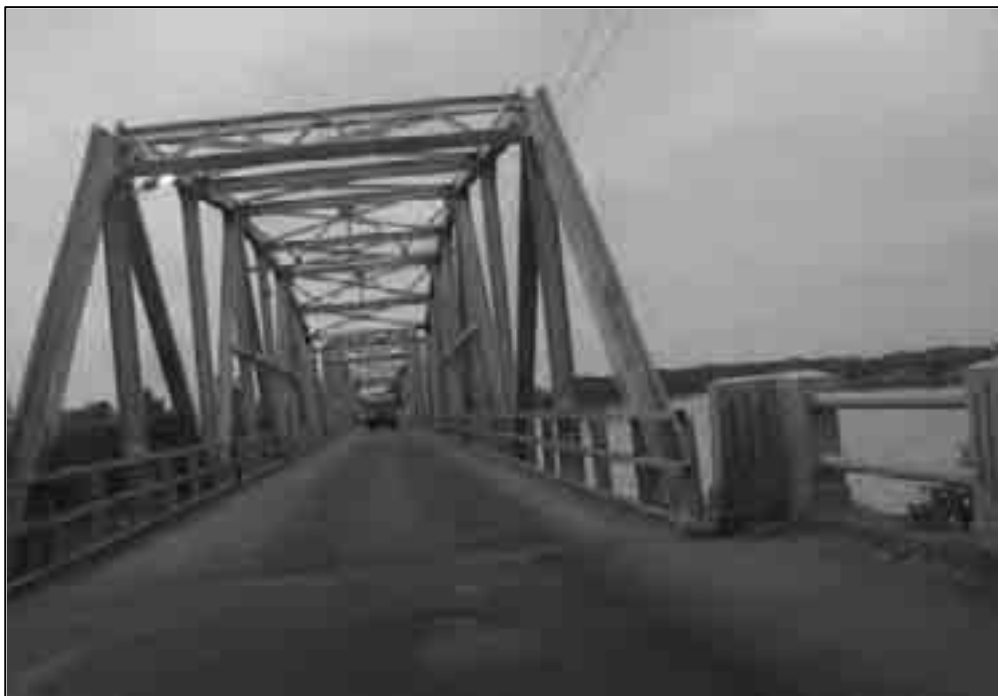
Figure 9-2: Existing bridge over the St George River
