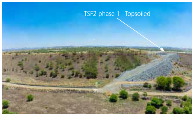
TSF 2 phase 1 – Topsoil and revegetation in progress
