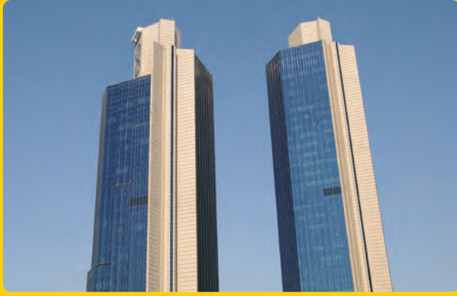
Sabancı Center – İstanbul, 1991
