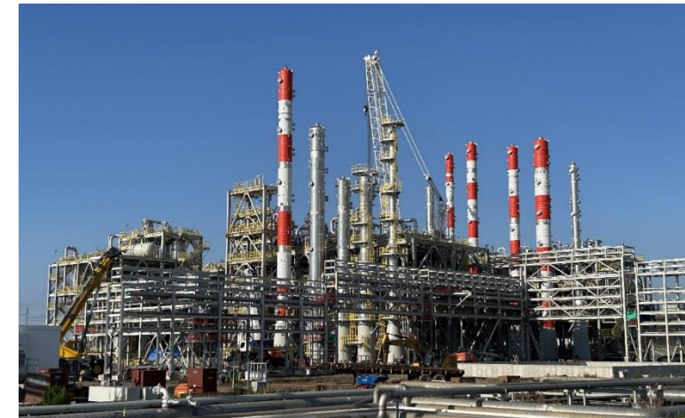
DMC & EMC plant under construction (as of May 2026)
