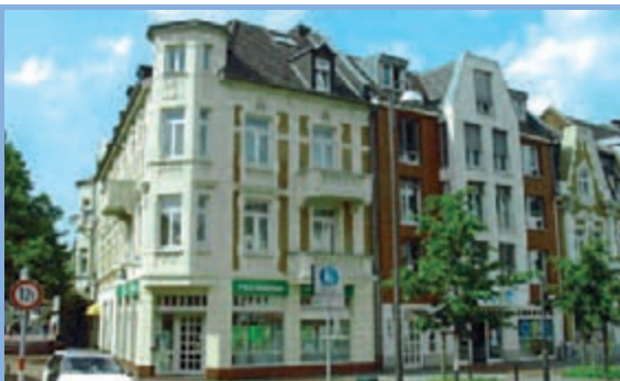
Office building, Bonn
