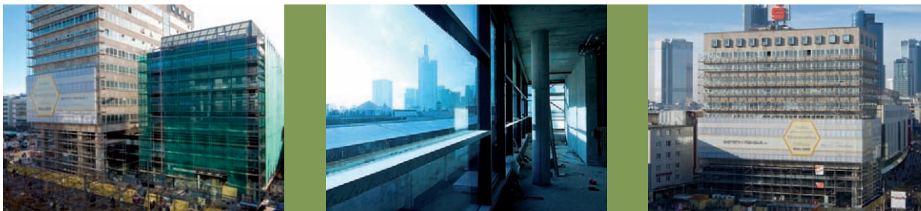
Frankfurt, Revitalisation and extension Bienenkorbhaus
