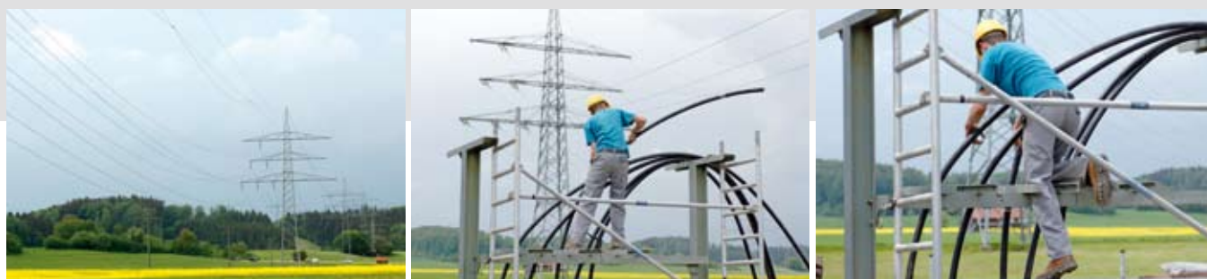
Installation: In a transformer substation, new 20 kV cables are fitted to a transformer.
