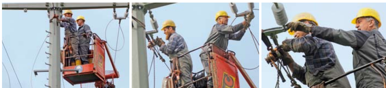
Installation: EnBW employees installing 20 kV electricity lines in the distribution network.
