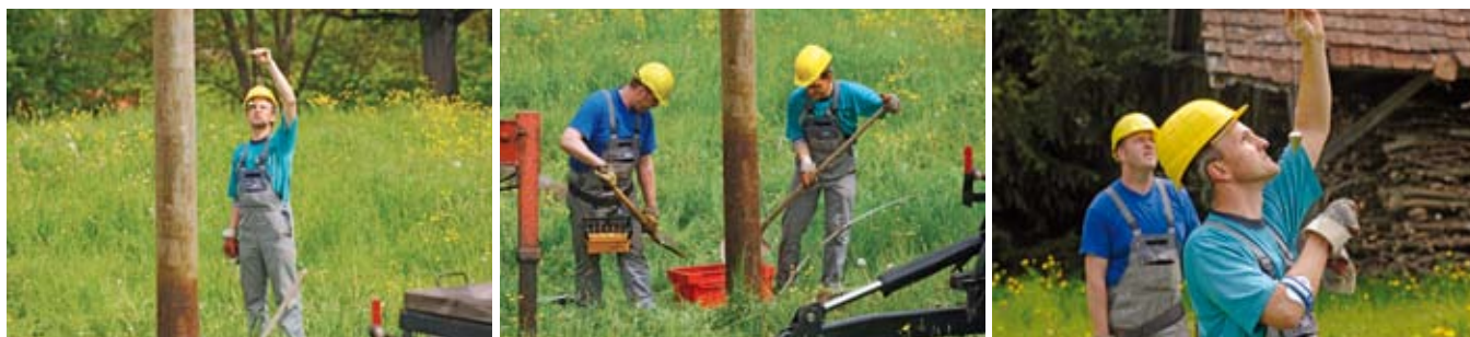
Infrastructure: EnBW employees make sure the masts are in good condition. New masts are carefully plumbed in.
