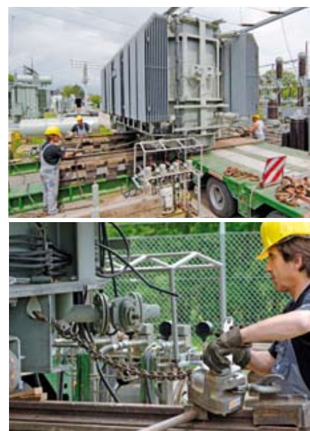
Modernisation: An old transformer is loaded onto an articulated lorry for removal.
