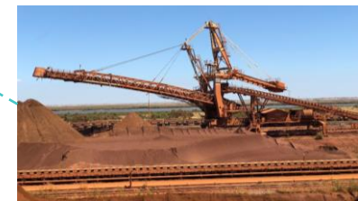
STK6: Stacker 6 upgrades
