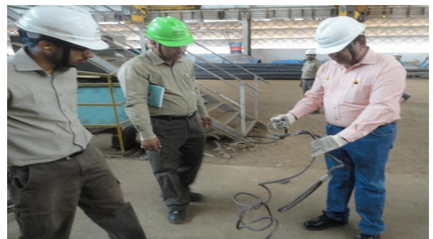
SAFETY AUDITS / INSPECTIONS
