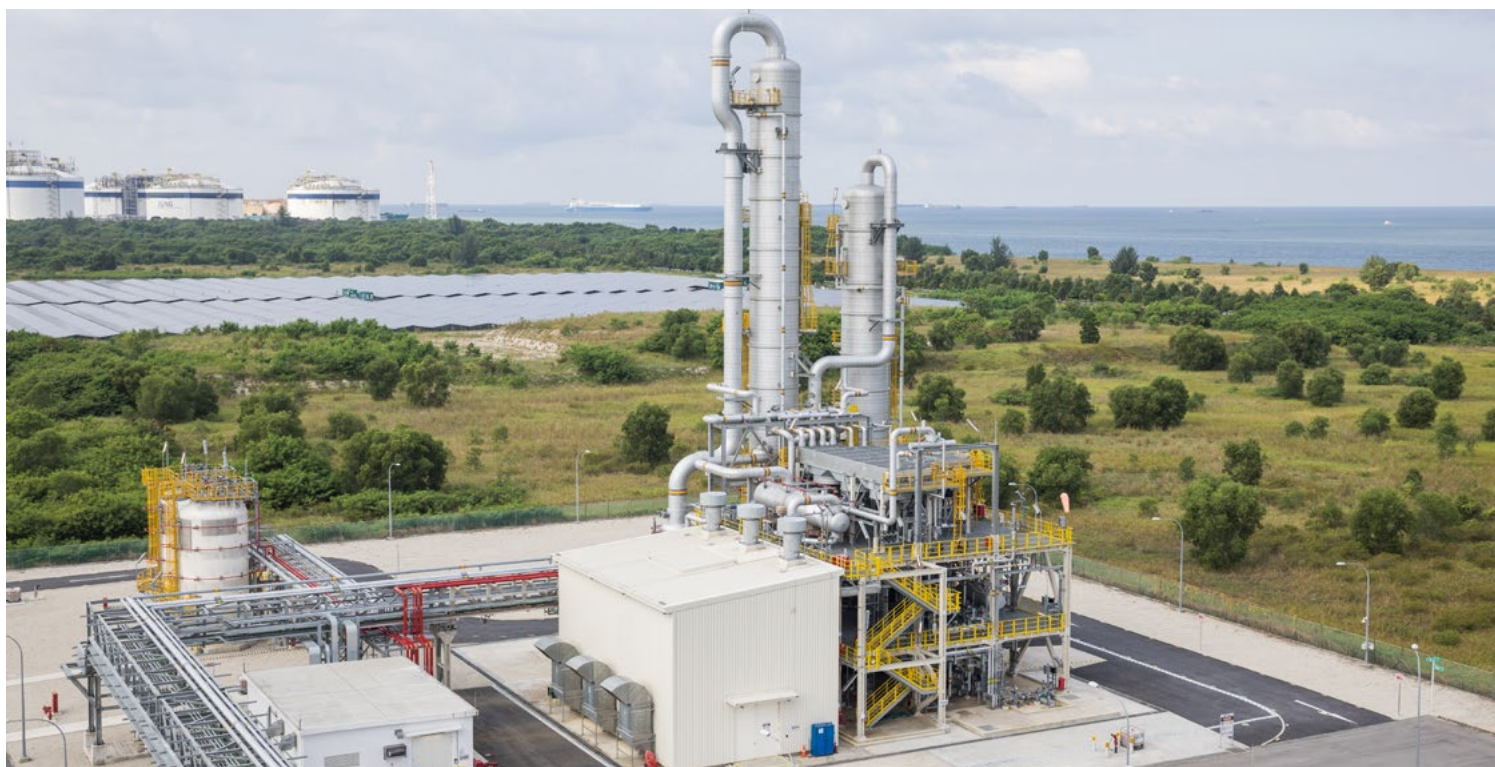
The new 100,000 metric ton production plant for alkoxides in Singapore.
