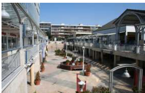
Centre commercial Elysée Village, Celle Saint Cloud (78)
