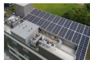
Solar power system installation
