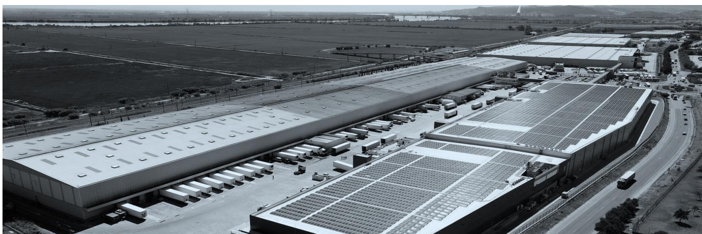
Aerial view of the recently expanded Azambuja distribution centre
