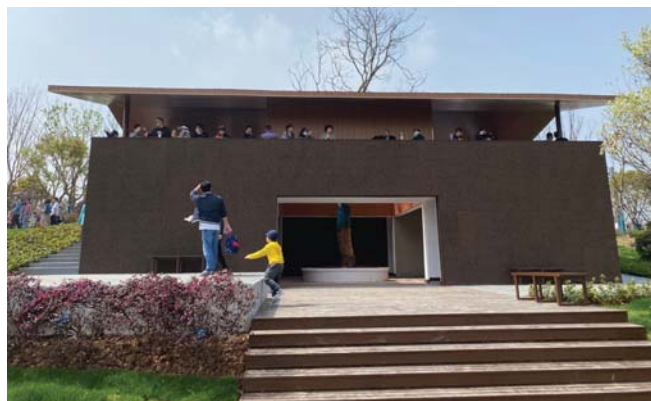
Amorim Cork Insulation's MDFacade Solution covers the Portuguese pavilion at a horticulture exhibition in China.
