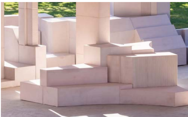
The cork used in the Serpentine Summer Pavilion responded to the challenge posed to Counterspace studio to build a temporary installation with a notable ecological character.
