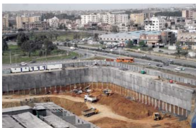
67 Peripheral Containment of the Basements of Air Algérie Headquarters Building
