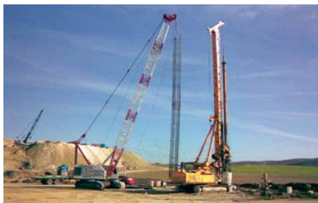
73 FERROVIAL / Piles and Jet-Mix, in viaduct La Motilla in Cuenca
