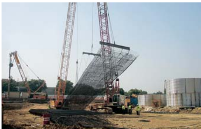
72 Sando / Bentonite Wall and Piles in the Interchanger of Mairena de Aljaraje
