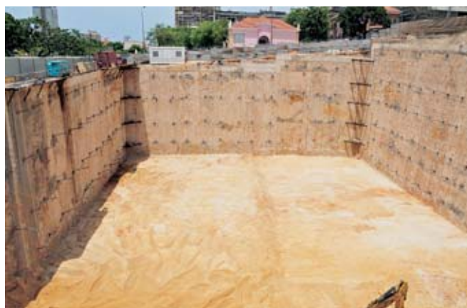
63 Bentonite Walls and excavation for Eight Basements in TORRES DO CARMO Building
