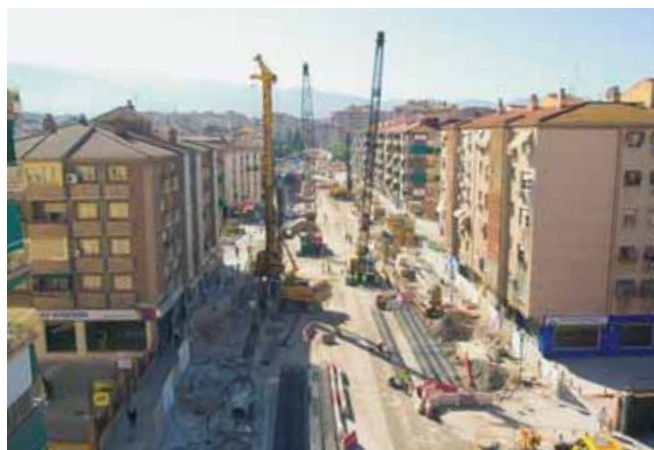
75 Ferrovial / 950 mm piles for the retaining walls of the channel of Metro de Granada
