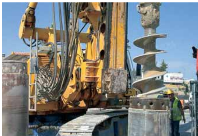
76 Ferrovial / 800 mm diameter pile wall, at Arroyo de los Migueles, on the A3 / Madrid motorway
