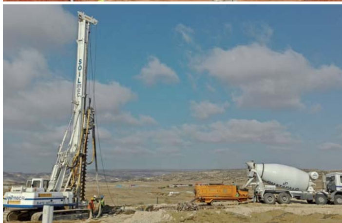
OMATAPALO - Indirect foundations of the building Talatona 2 Luanda | Angola
