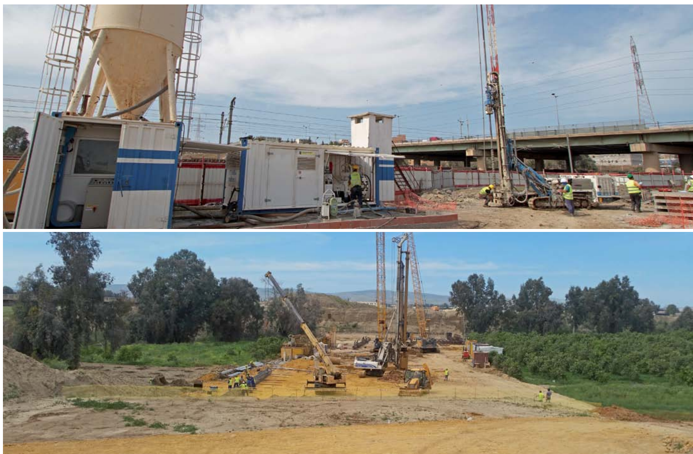
A.P.P.L. - Micro-pile and jet grouting work Algeria
