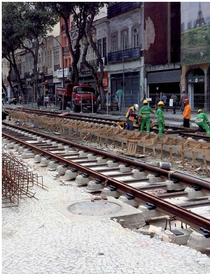
VLT Carioca - Installation of surface light rail transit track Rio de Janeiro | Brazil
