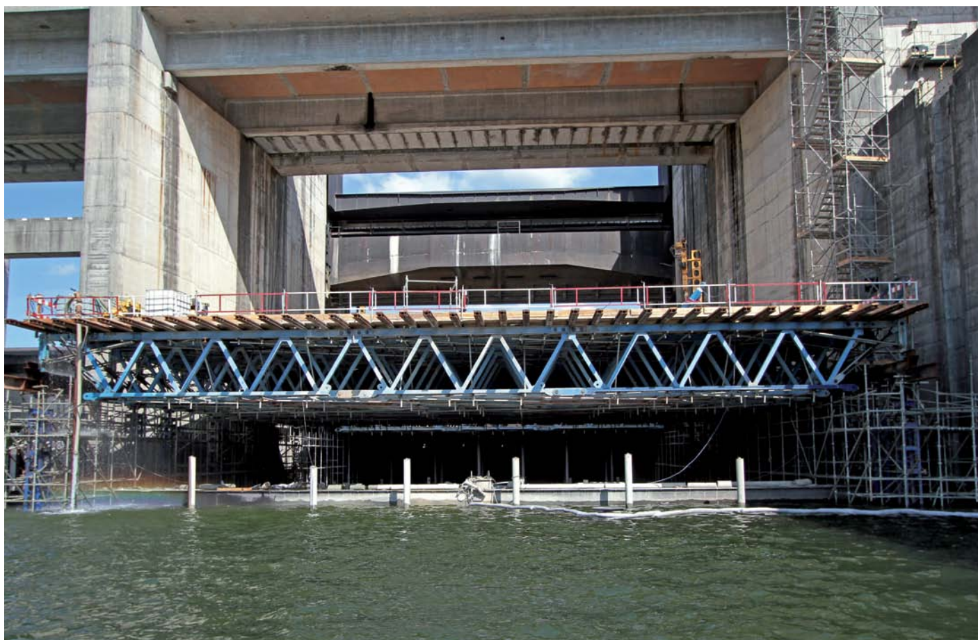
Crestuma Dam - Design and assembly of a platform for the execution of geotechnical work Porto | Portugal
