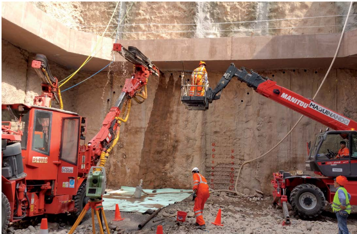
Construtor M2 Lima Consortium – Excavation and coating of two galleries in Lima Metro Lima| Peru
