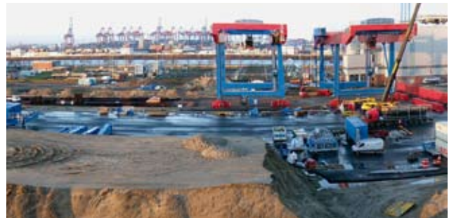
Rail gantry cranes being installed at Tollerort on-dock container rail terminal.
