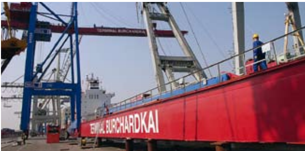
Erection of a container gantry crane on Burchardkai.
