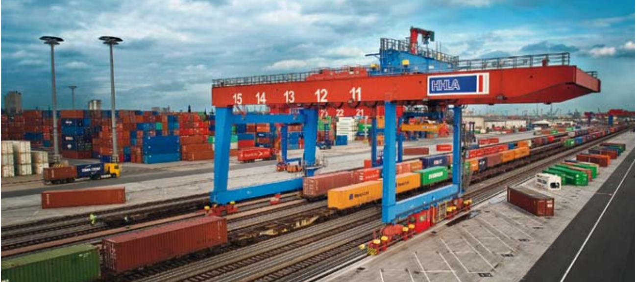
The on-dock container rail terminal at Burchardkai opened in 2006: cranes working on complete block trains on eight tracks, each over 700 metres long.
