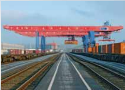
The rail terminal with seven sidings ensures that more goods can be transported by rail, which is better for the environment. Block container trains can be marshalled directly without shunting.
