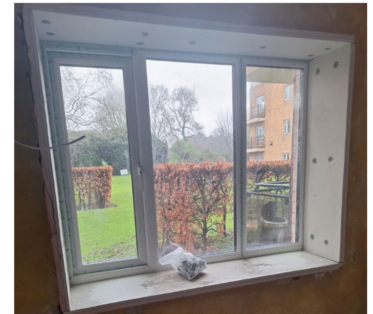
Thick external wall insulation and double-glazing upgrade to reduce the amount of energy needed for heating.
