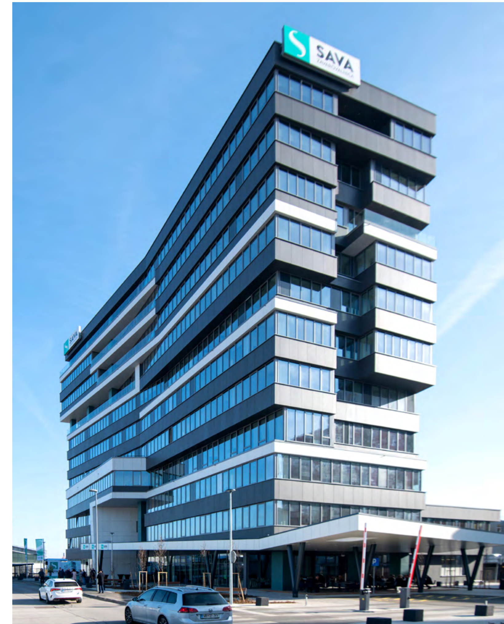
Zavarovalnica Sava’s (SVN) investment in an energy-efficient office building in Maribor, the new head offices of six Group companies.
