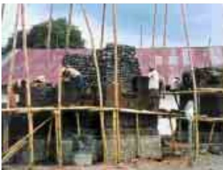
Scaffolding made from bamboo is tried and tested.
