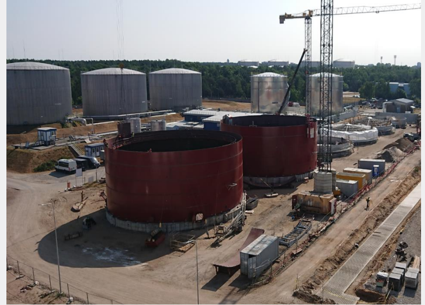
LFO 2 x 10 000 m3 and 4 x 5 000 m3 tanks installation - Earth works and foundations installation works have been done for all tanks.
