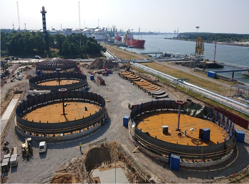
LFO 6 x 20 000 m3 tanks installation - earth works and foundations installation works have been done for 4 out of 6 tanks.
