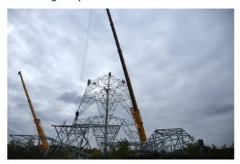
The construction works of the Ostrovu Mare - ETG (new line) 220 double-circuit OHL 220, which will contribute to the discharge of energy produced in the Porţile de Fier 2 hydropower plant, are at an advanced stage of execution. The line is about 31 kilometers long, has 105 poles and crosses the territory of 5 administrative territorial units in Mehedinţi County.
