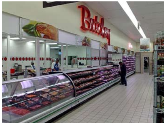
Beijer Ref's company in South Africa, Metraclark, delivers refrigeration and freezing systems to the Checkers grocery chain.
