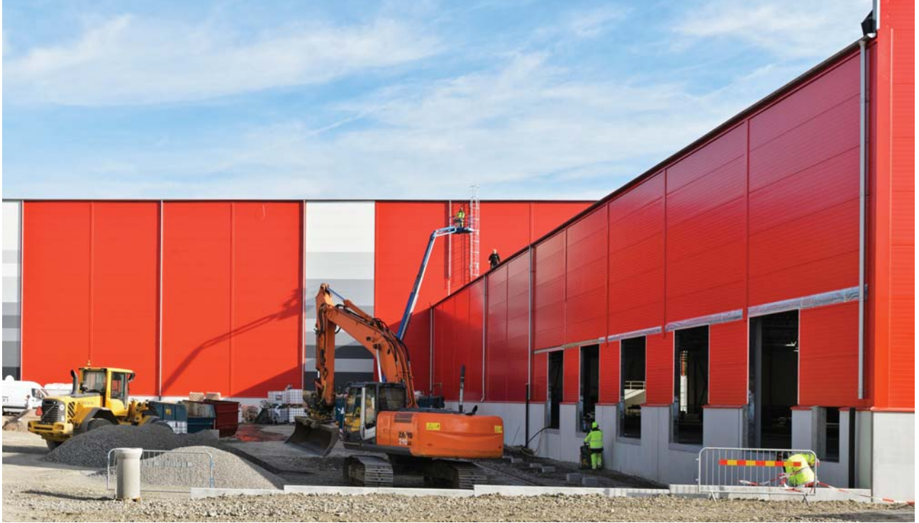
In Berga, Helsingborg, a logistic property of 9,700 sq.m is under construction.
