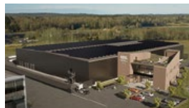
Aseby 1:5 Gothenburg ONGOING New construction, pub. sector Investment: SEK 301 M
