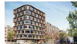
GreenHaus Helsingborg COMPLETED OR FULLY/PARTIALLY OCCUPIED New construction, office
