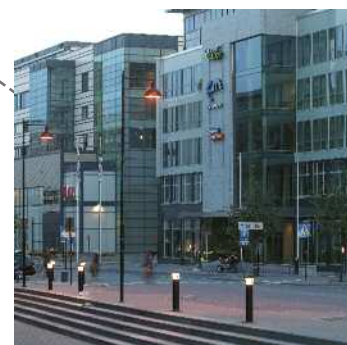
Fräsaren 11 , Solna Business Park.
