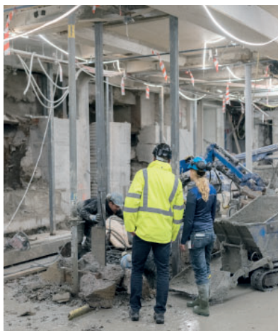
Reinforcing the foundations at the NK department store in Gothenburg.
